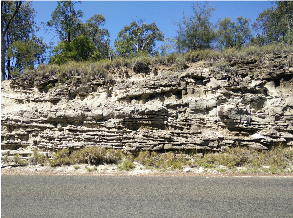
Plate 4b: Orallo Formation central part of road cutting.
